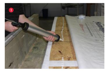
Apply DuPont™ Residential Sealant, or recommended sealant, along the top/bottom of the wall approximately 2 to 3" from the edge. Press the Tyvek® WRB into the sealant using firm hand pressure or a J-roller. This will temporarily hold the Tyvek® WRB in place in prior to step 2.
