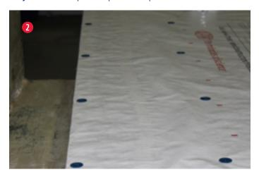
Fasten the Tyvek® WRB to the studs as instructed in the DuPont™ Tyvek® Water-Resistive and Air Barriers Installation Guidelines For Buildings Less Than 5 Stories and Low-Rise Multi-Family Residential Buildings Less Than 6 Stories.
