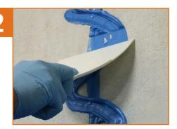
Spread the SOPREASEAL Liquid Flashing membrane with a trowel to acheive a monolithic flashing at a minimum of 20 wet mils, free of voids or pinholes. Allow product to skin prior to spraying.
