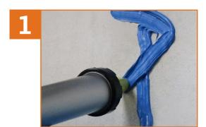
Prior to spraying SOPRASEAL LM 204 VP, prepare all sheathing joints by applying a thick monolithic bead of SOPREASEAL Liquid Flashing into the joint. Create a zigzag pattern over the joints with a minimum of 2 inches of coverage.
