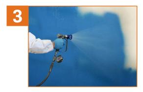
Apply SOPRASEAL LM 204 VP to the desired thickness directly to the prepared substrate.
