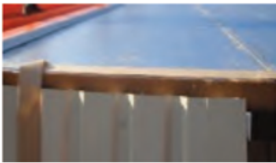
DuPont™ Thermax™ Insulation with Weathermate™ Flashing Applied
