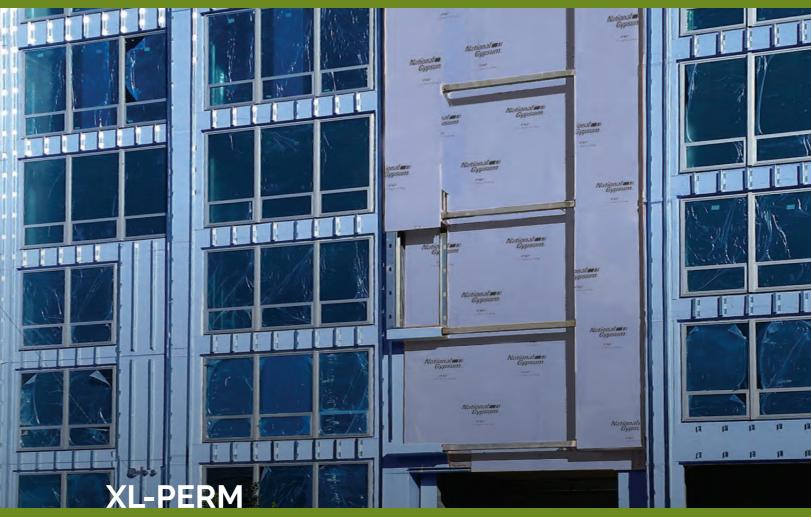
AIR, VAPOR AND WATER RESISTIVE BARRIER SYSTEM
