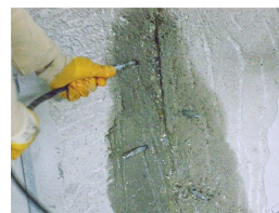
Hose set coupling to installed mechanical packer.
