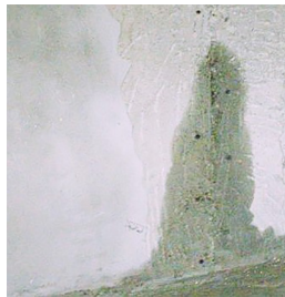
Staggered port placement on vertical crack.
