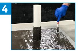
Once cured, apply a final coating of ALSAN Flashing at a rate of two gallons per 100 ft² to the pipe and field, extending approximately 1" past the previous coat.
