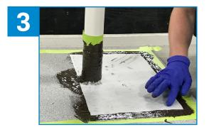
Apply ALSAN Flashing to the taped off field area at a rate of two gallons per 100 ft², lay fleece into the first coat and apply second coating of ALSAN Flashing. Remove the tape.
