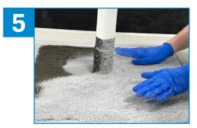
While it is not required, if desired, granules may be broadcast into the final coat of ALSAN Flashing to match the cap sheet.
