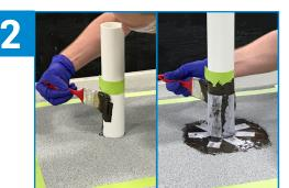
Apply ALSAN Flashing liberally with a brush at a rate of two gallons per  $100 \, \mathrm{ft^2}$  to the pipe, wrap the fleece around pipe or penetration and coat with an additional layer of ALSAN Flashing.
