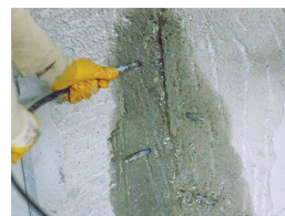
Hose set coupling to installed mechanical packer.
