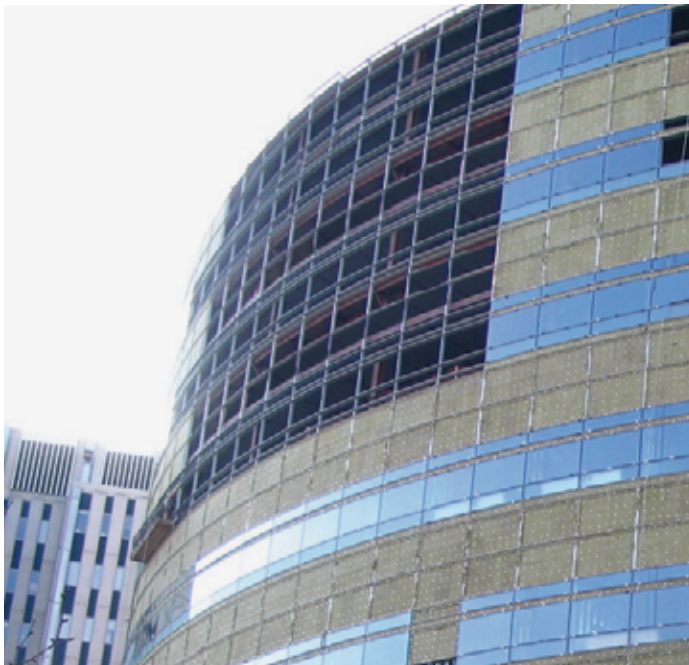
In addition to superior sound absorption properties, ROCKWOOL CURTAINROCK® and ROXUL SAFE™ are frequently specified for a variety of commercial curtain wall applications.
