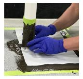
11. Apply fleece into wet ALSAN Flashing and coat the full field area with ALSAN Flashing at a rate of 2 gallons per square. Ensure that the fleece is completely saturated and there are no voids or dry areas.
