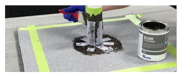
8. Apply ALSAN Flashing to ½ of the field area at a rate of 2 gallons per square, look for similar coverage as the first application to the pipe and no dry spots.
