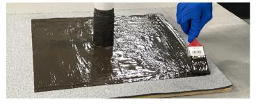
Apply the second coat of ALSAN Flashing to pipe and field after first coat cures approximately 1¼" past the previous application at a rate of 2 gallons per square.
