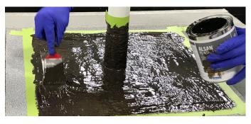
Remove tape around pipe and field and let dry 24 to 48 hours (curing time may vary with temperature and humidity).
