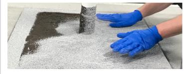
14. ALSAN Flashing may be left unprotected. Though not required, granules may be broadcast into flashing until refusal. Wait for coat to dry and then brush off remaining granules.
