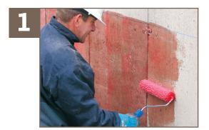
Prime the substrate with ELASTOCOL Stick, ELASTOCOL Stick Zero or ELASTOCOL Stick  $H_2O$ .
