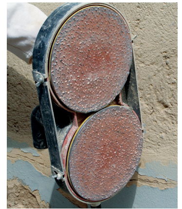
Removing old plasters
