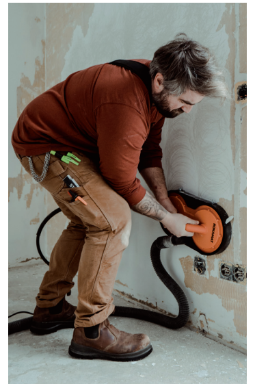
Removing old paint
