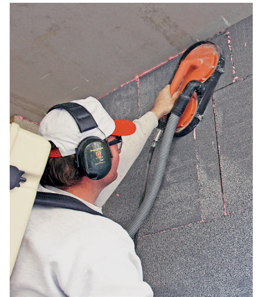
Grinding EIFS and ETICS boards
