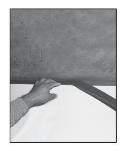
Foam is simple to install for head of wall applications. Compress the Blaze Foam into the joint between the top of the wall and bottom of the deck so that the intumescent strip is facing the wall surface. Blaze Foam can be recessed into the joint or installed flush with the outside surface of the wall. Joints are butted together. No mechanical fastening of Blaze Foam is required.
