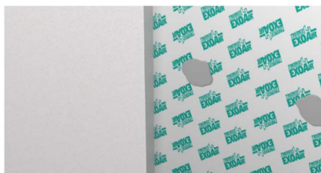
Ref 2 – Insulation installed
