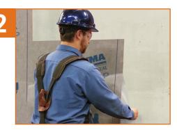
Gradually peel off the remaining silicone release film, making sure the membrane adheres completely to avoid air pockets and wrinkles.
