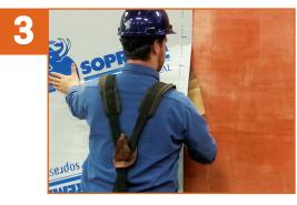
Gradually peel off the remaining silicone release paper, making sure the membrane adheres completely to avoid air pockets and wrinkles.
