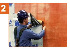
Peel off the top portion of the silicone release paper and adhere the membrane to the substrate, making sure the membrane is well aligned.
