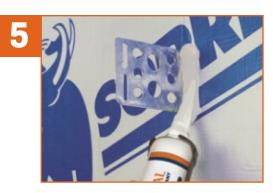
Use SOPRASEAL Sealant to seal around details, reverse laps and critical areas. For window openings, use a compatible sealant.
