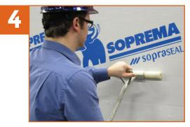
Use a roller to apply pressure over the entire surface of the membrane to ensure uniform adhesion to substrate.
