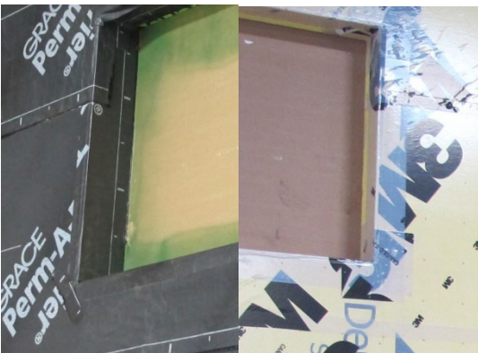
Figure 4: Window Penetration Detail
