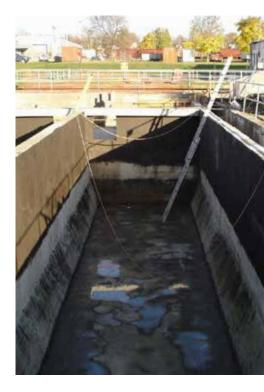
CEM-KOTE FLEX CR is primarily used for waterproofing and protection of concrete structures exposed to sulfuric acid (generated by microbiological oxidation of hydrogen sulfide).
