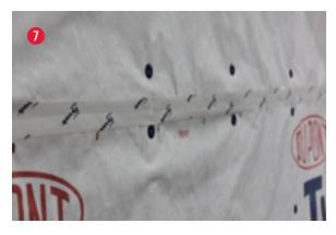
7. Tape all seams with **DuPont™ Tyvek® Tape**, and verify sealant "connection" between wrap and wood. Use hand pressure or j-roller as necessary to ensure a good bond.
