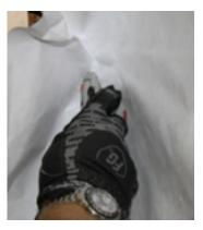
Install the Tyvek® WRB onto framing and tuck edges tightly into sealant and corners of framing as shown above. Use firm hand pressure or J-roller to ensure a positive bond to sealant. Cut excess Tyvek® WRB.
