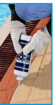
Seal all cracks and joints with DECK-O-SEAL two-part, elastomeric, polysulfide-based joint sealant. It is ideal for sealing joints in and around swimming pools, and is applicable for both interior and compression or elongation.
