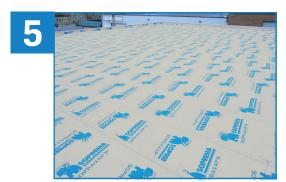
SOPRAVAP'R may be left in place during construction. When left exposed to precipitation, positive slope and adequate drainage is required. The effects of weathering may vary based upon local climate and project conditions. Cover as soon as possible to limit exposure to UV and construction traffic. Not recommended for use as a temporary roof assembly.
