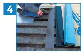
At the end of each roll, install a sheet metal plate (6 x 42 in /  $15 \times 106$  cm) to support the end lap between deck ribs. Ensure 6 in (15 cm) end laps are maintained during installation.
