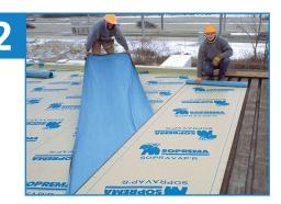
Once SOPRAVAP'R is in place, while holding the sheet tight, remove the silicone release film by pulling diagonally.
